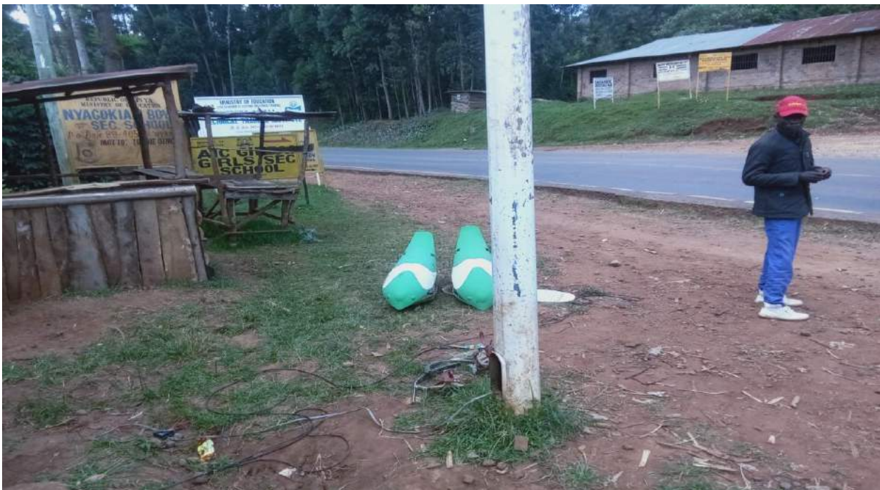
Repair of Nyagokiani junction streetlights
