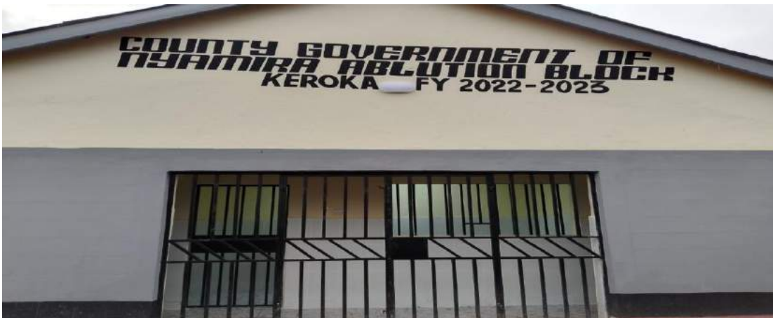
Keroka ablution block
