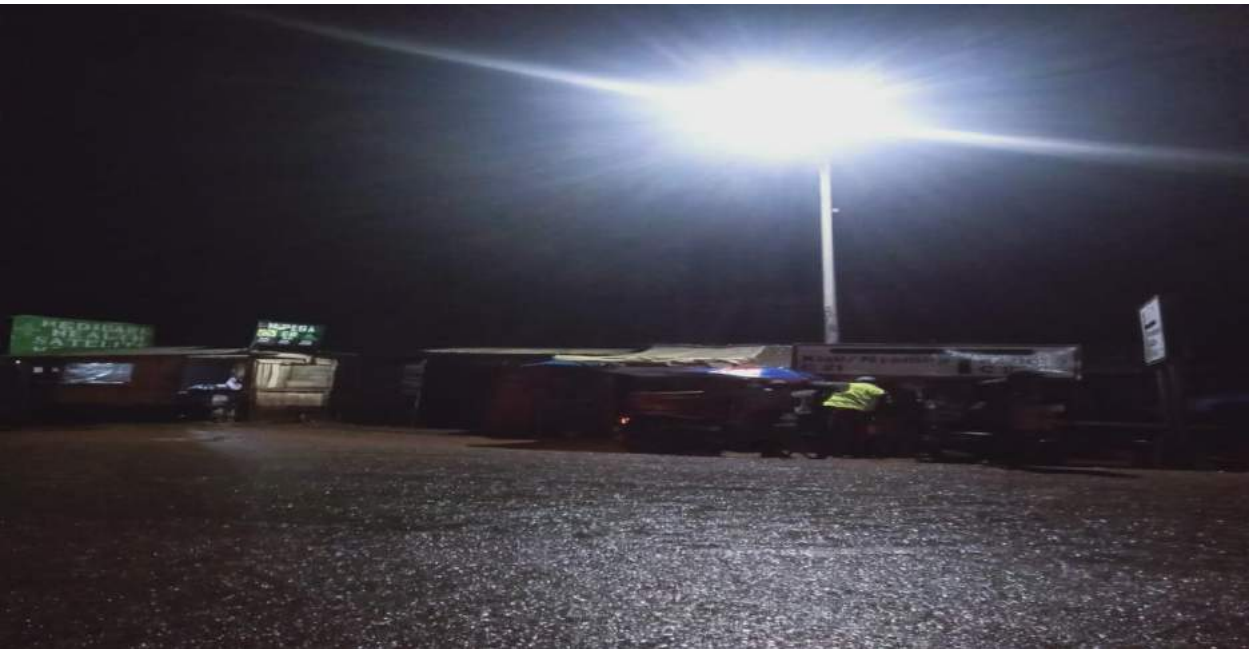
Repair of Kebirigo – Nyamira Stage streetlights at Kebirigo
