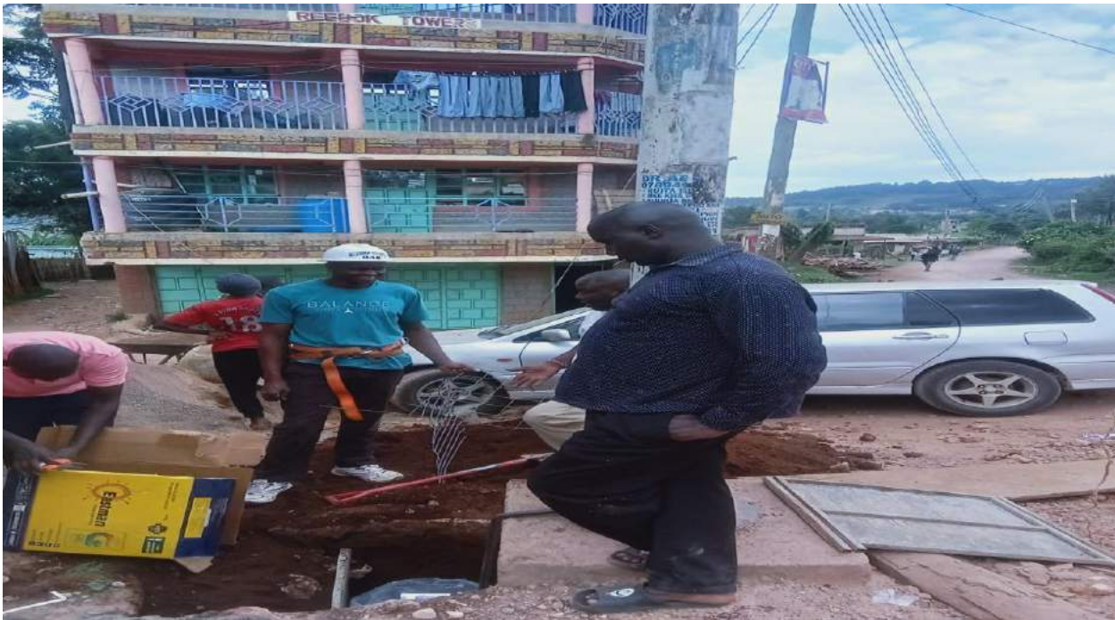
Repair of Keroka Markwet streetlight at Roy Resort Gate
