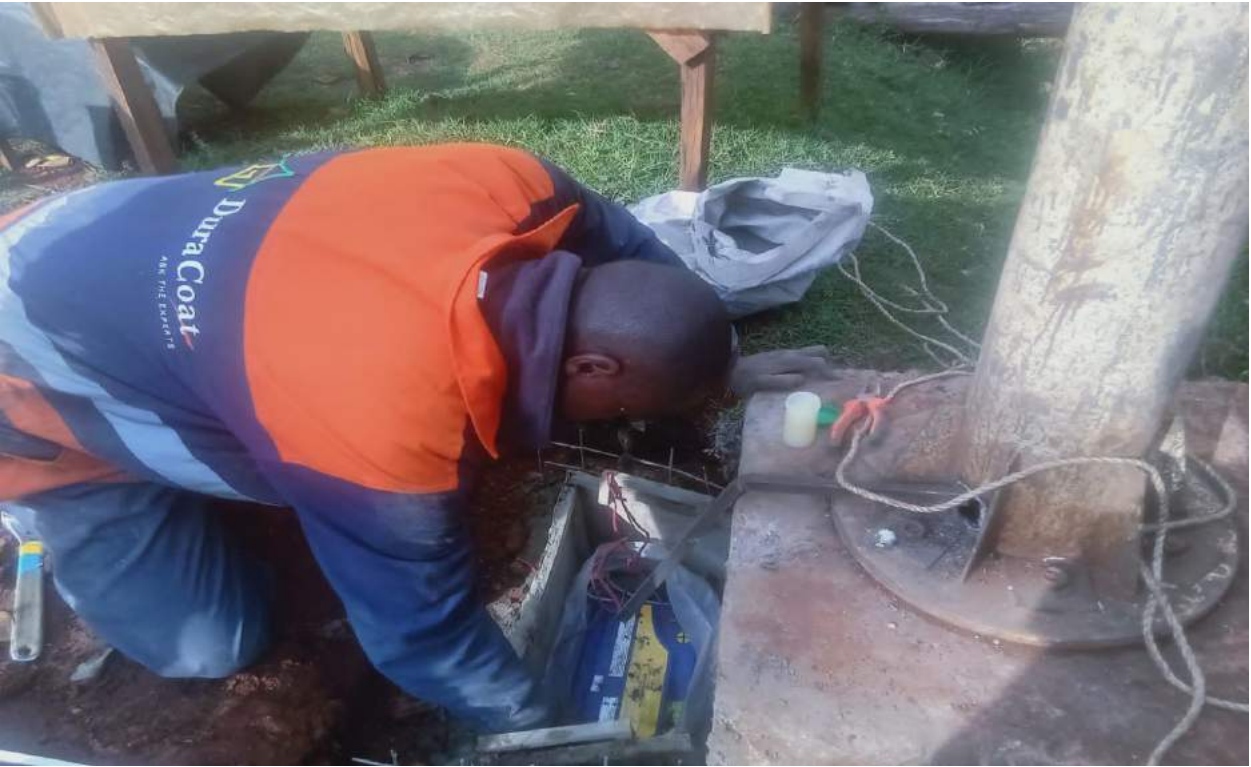
Repair of streetlights at Sironga Buying Centre in Bogichora Water
